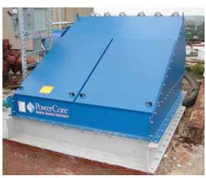
**CPV-12 - Cement silo bin vent conveyor** 3,700 cfm (6,285 m<sup>3</sup>/h)
